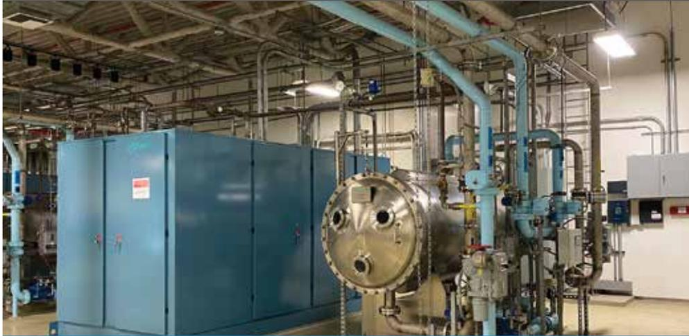
**Photo:** An ozone generator at the R.M. Levy Water Treatment Plant. Inside the generator, electricity splits oxygen molecules ( $O_2$ ) and forms ozone ( $O_3$ ), which we use to disinfect water during the treatment process.
